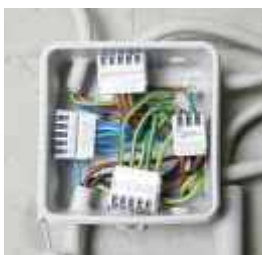
Free Floating connectors suitable for smaller size Junction Boxes
